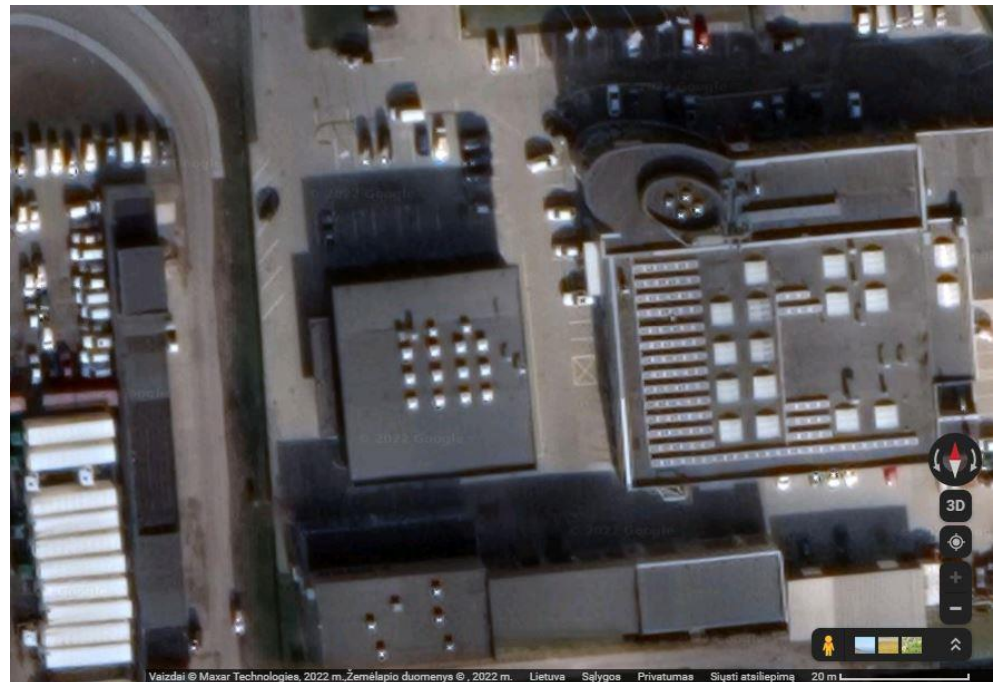
Figure 10. The view of the as-built auto repair shop. The photo was taken using the Google maps tool on 6 June 2022.
