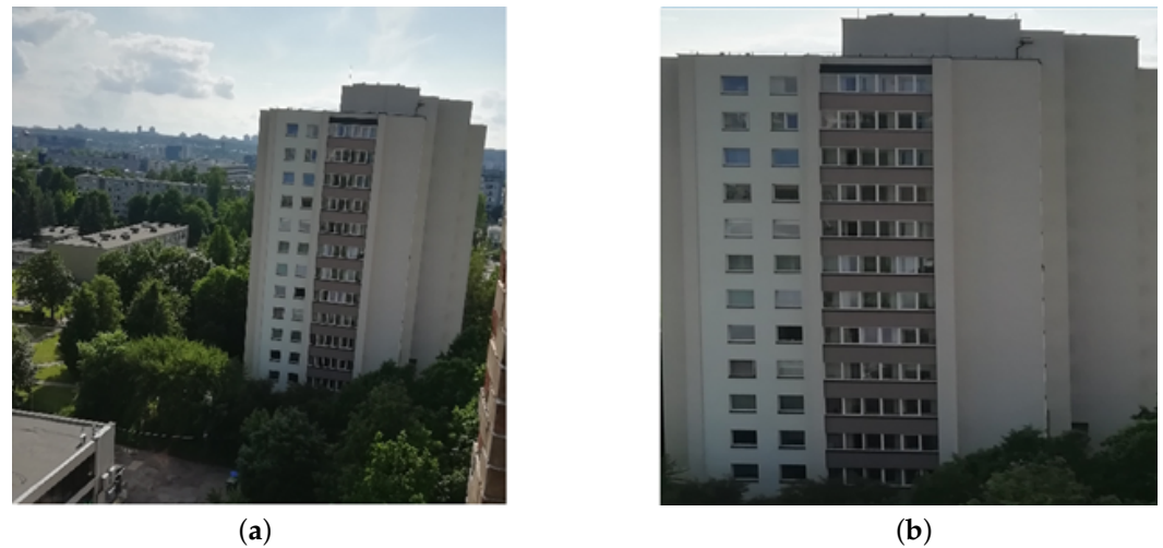
Figure 6. Example of building façade detection: (a) the original image obtained, and (b) the transformed image in order to have only a view of the façade exactly from the front.
