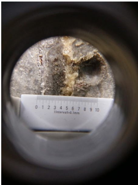
Fig. 7. Crack completely healed after 21 days of being exposed to constant water pressure.
