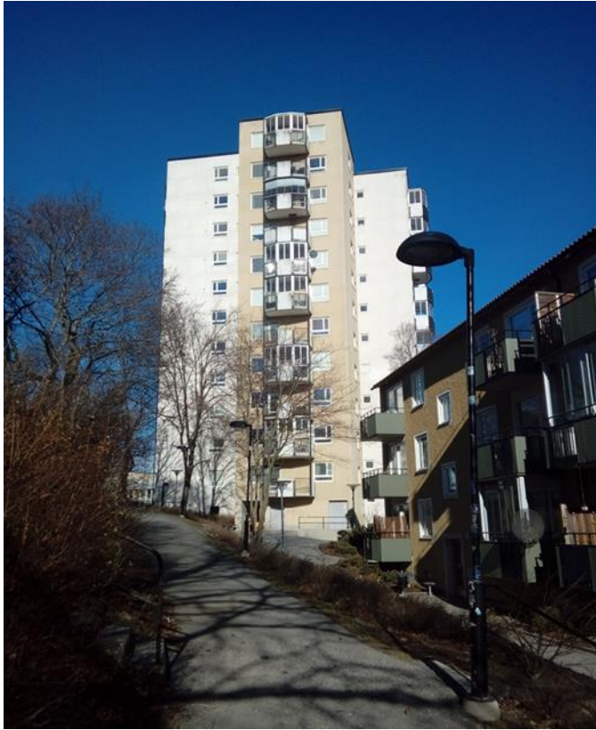
Fig. 24. Vällingby: integration of architecture and natural topography of the site
