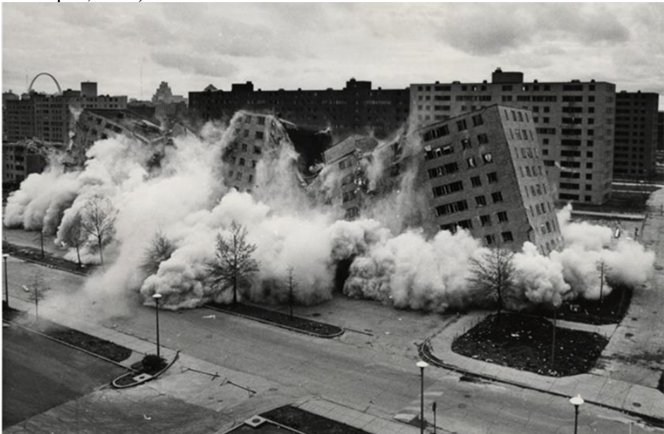
Fig. 6. The demolition of Pruitt-Igoe (© St. Louis Post-Dispatch)
