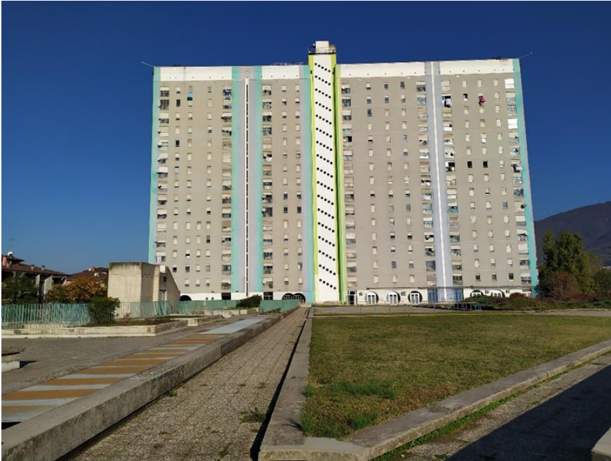
Fig. 48. The Cimabue tower (photo by the author)
