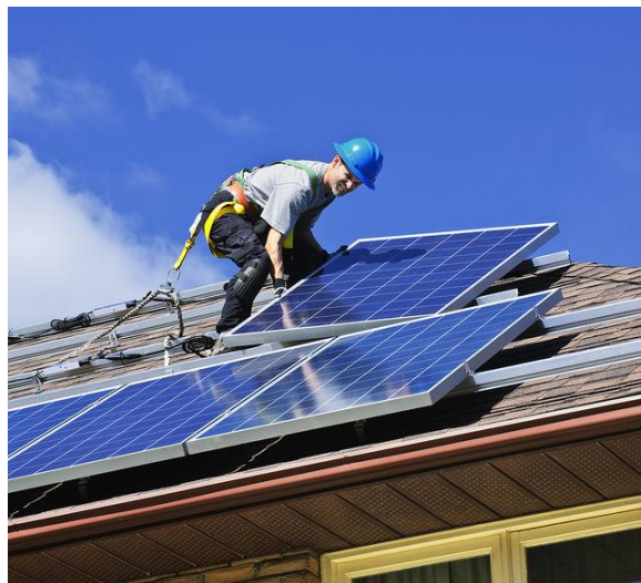
Fig. 19 Photovoltaic Panel installation by evergreen solar.
