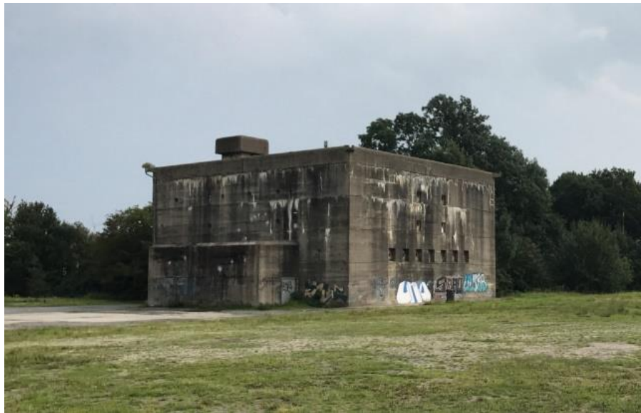
Fig. 24 Prussian Navy Bunker at Wilhelmshaven, Germany. (Block, 2021)
