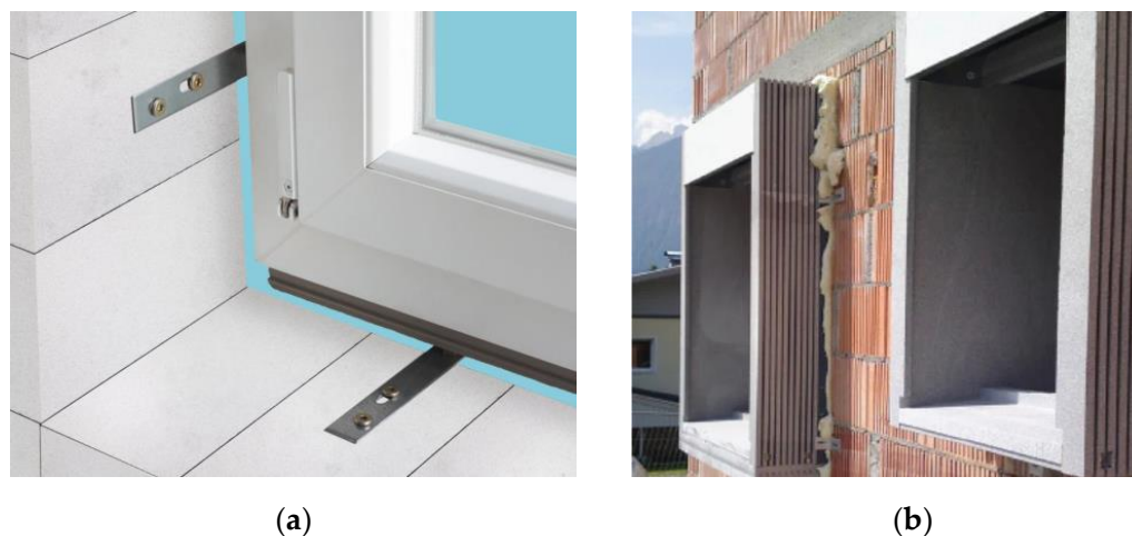
Figure 2. System of window installation in the insulation layer: (a) on anchor brackets [27]; (b) on chipboard frame [28].
