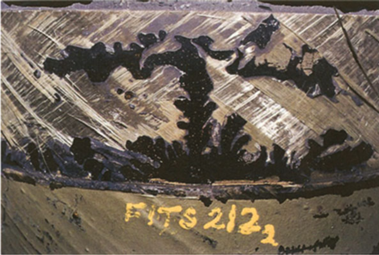
Fig. 3.55 Void in the adhesive caused by premature handling of the joint before the adhesive cured (da Silva et al. 2018)
