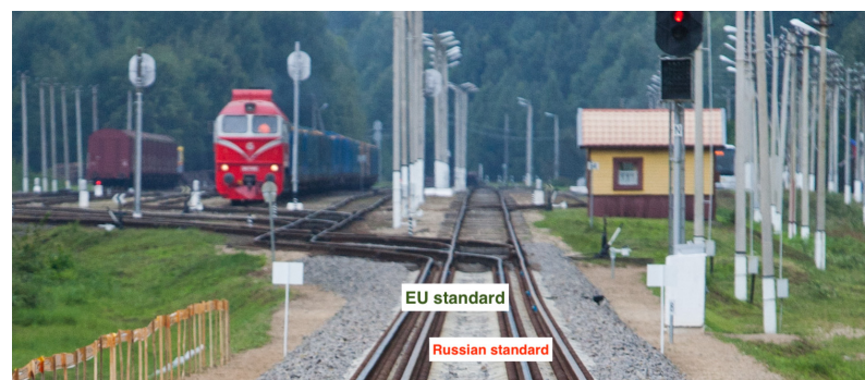
Figure A10. Difference in the width of EU and Russian rail tracks.
